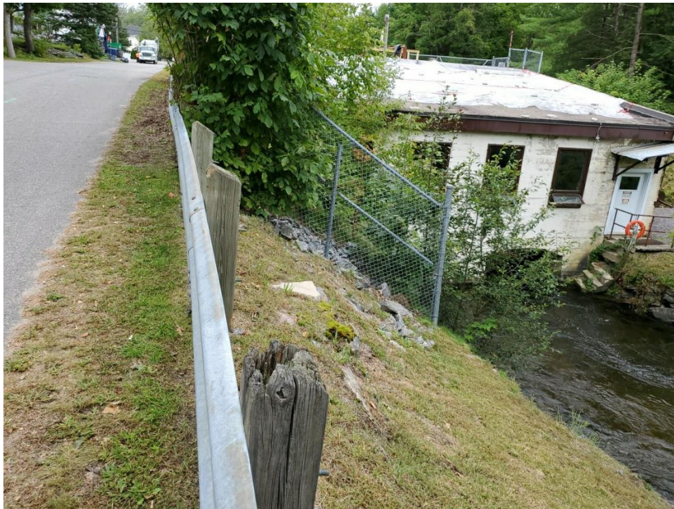
Photo 4: North Slope with powerhouse and tailrace in background on right. Note abrupt slope change where gabion basket wall exists at break in slope.
