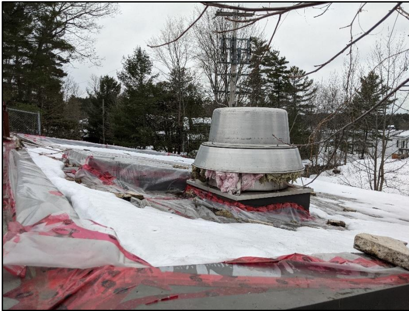
Figure 4: Unfinished Roof Surface
