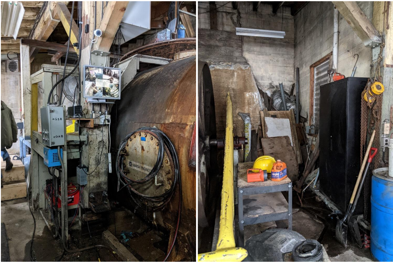
Figure 9: Station Cleanliness and Concrete Degradation/Oil Saturation
