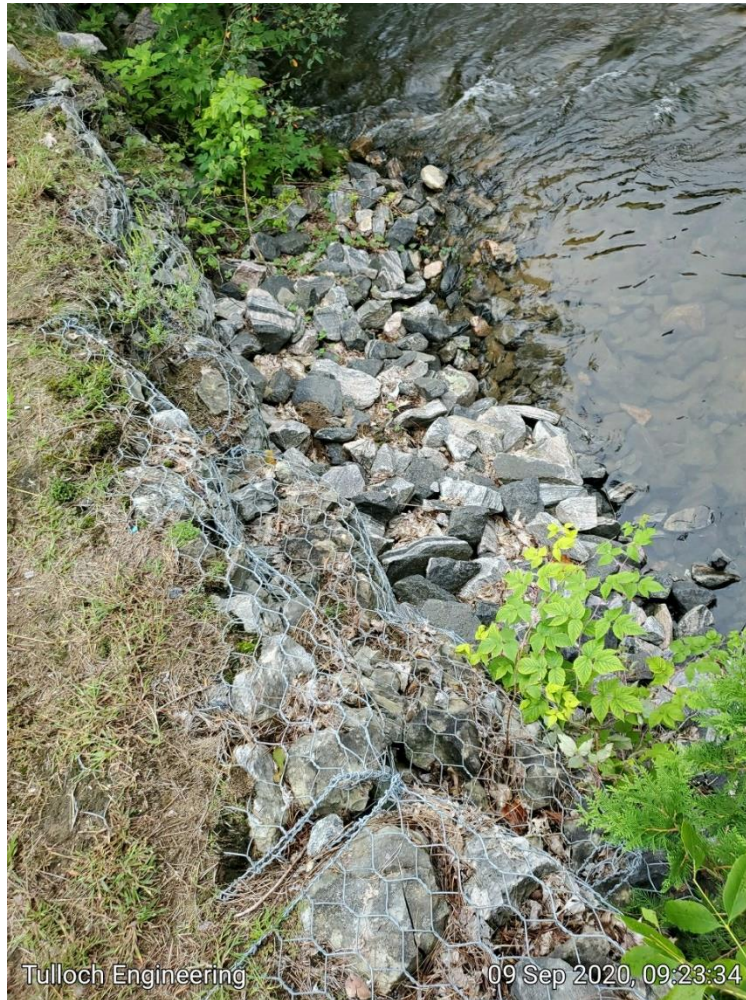
Photo 5: Gabion wall at toe of North Slope. Note rockfill located at toe of gabion wall above tailrace water level.
